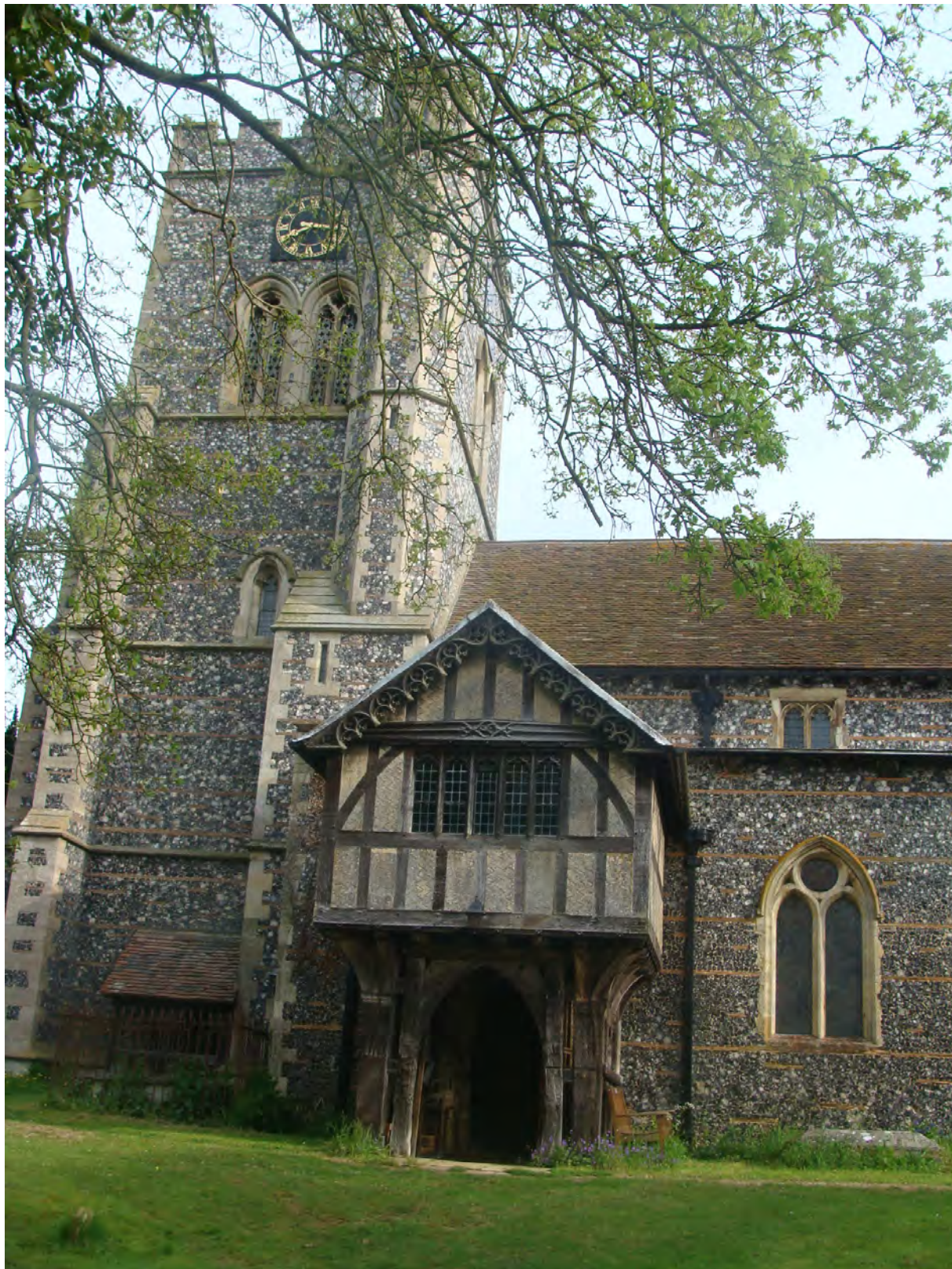
Picture 1.10 Radwinter church, note similarity of porch with Nesfield's original sketch, see Picture 1.5 above
