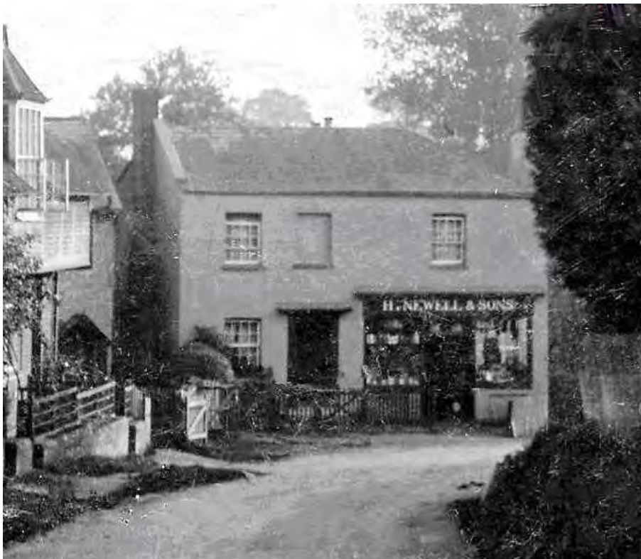
Picture 1.1 Traditional village shop and residence early/mid 20th century
